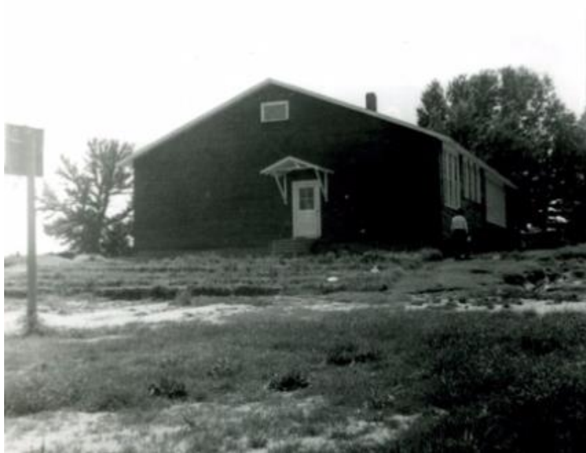
Figure 3: Isaac School, photograph 1955 taken as part of a statewide school survey mandated by the Legislature. This picture shows that the school never had the half-width porch that was shown in the standard Rosenwald Plan #3-B.
