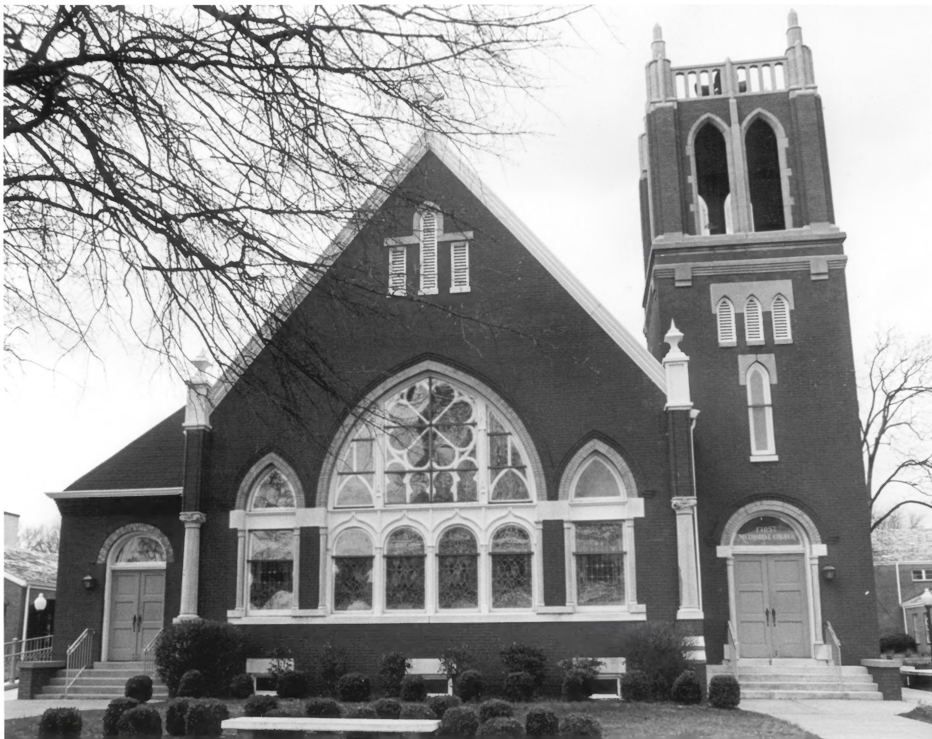
First Methodist Church, Photo 1 of 11
