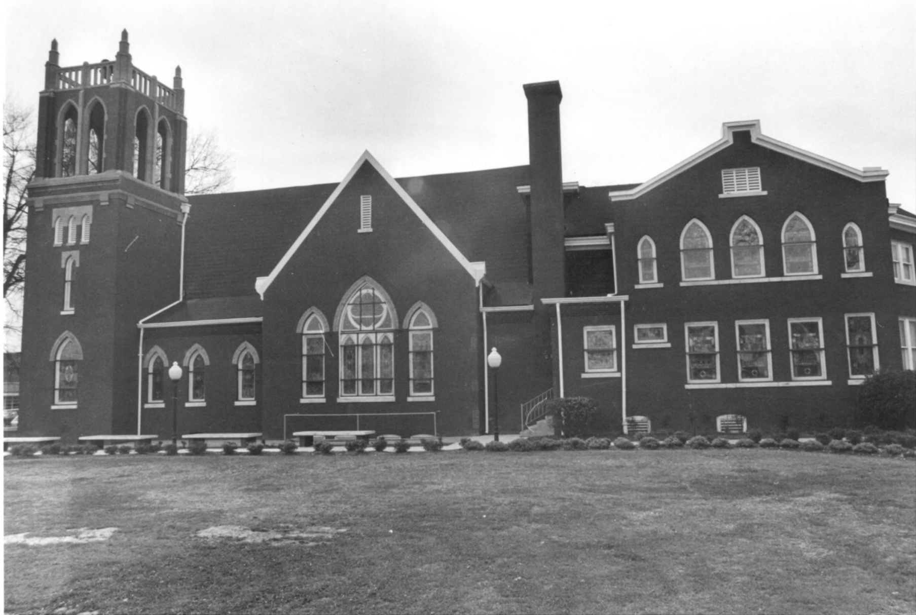
First Methodist Church, Photo 4 of 11
