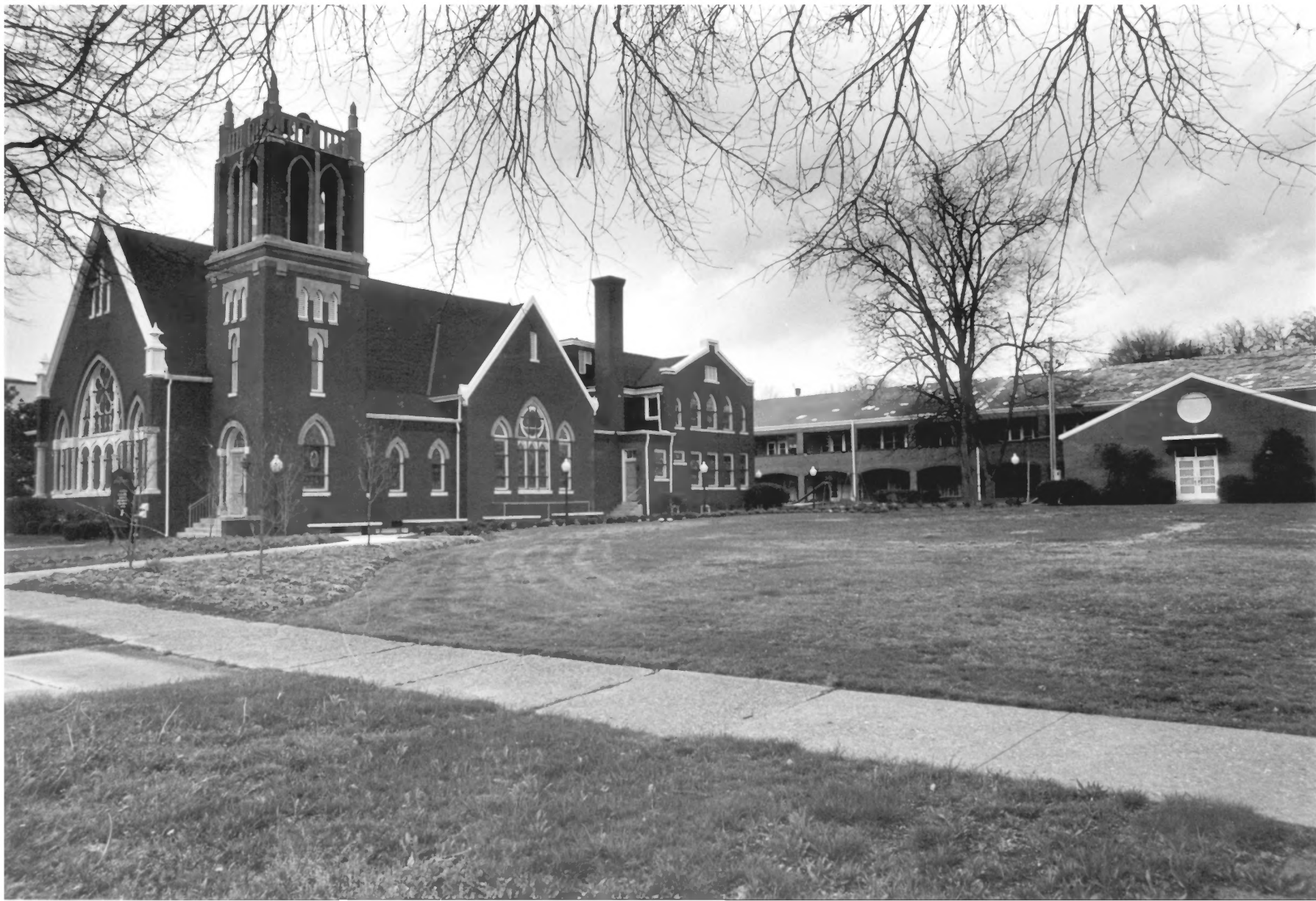
First Methodist Church, Photo 2 of 11
