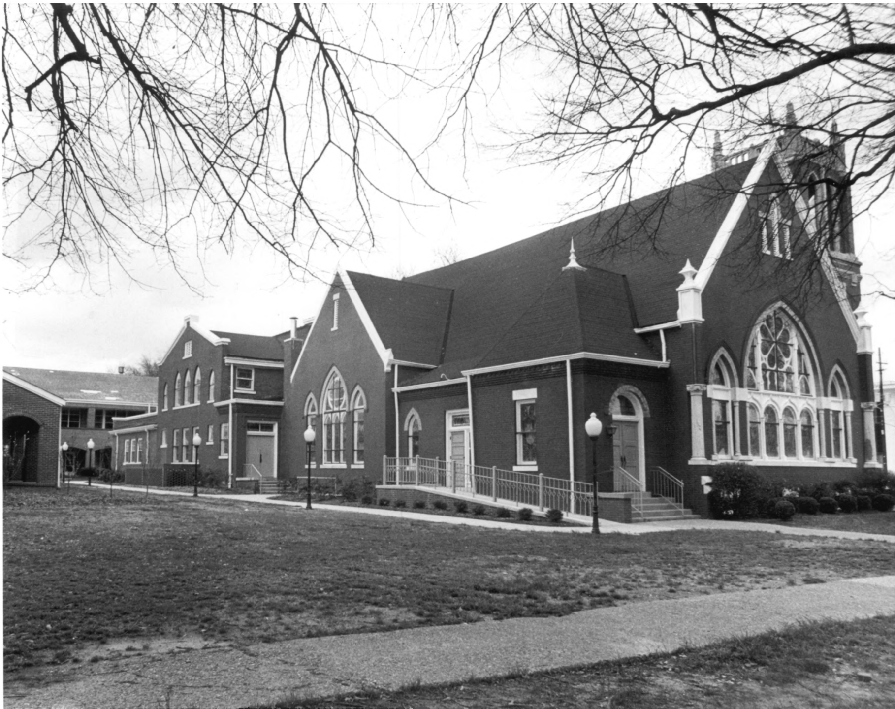
First Methodist Church, Photo 3 of 11
