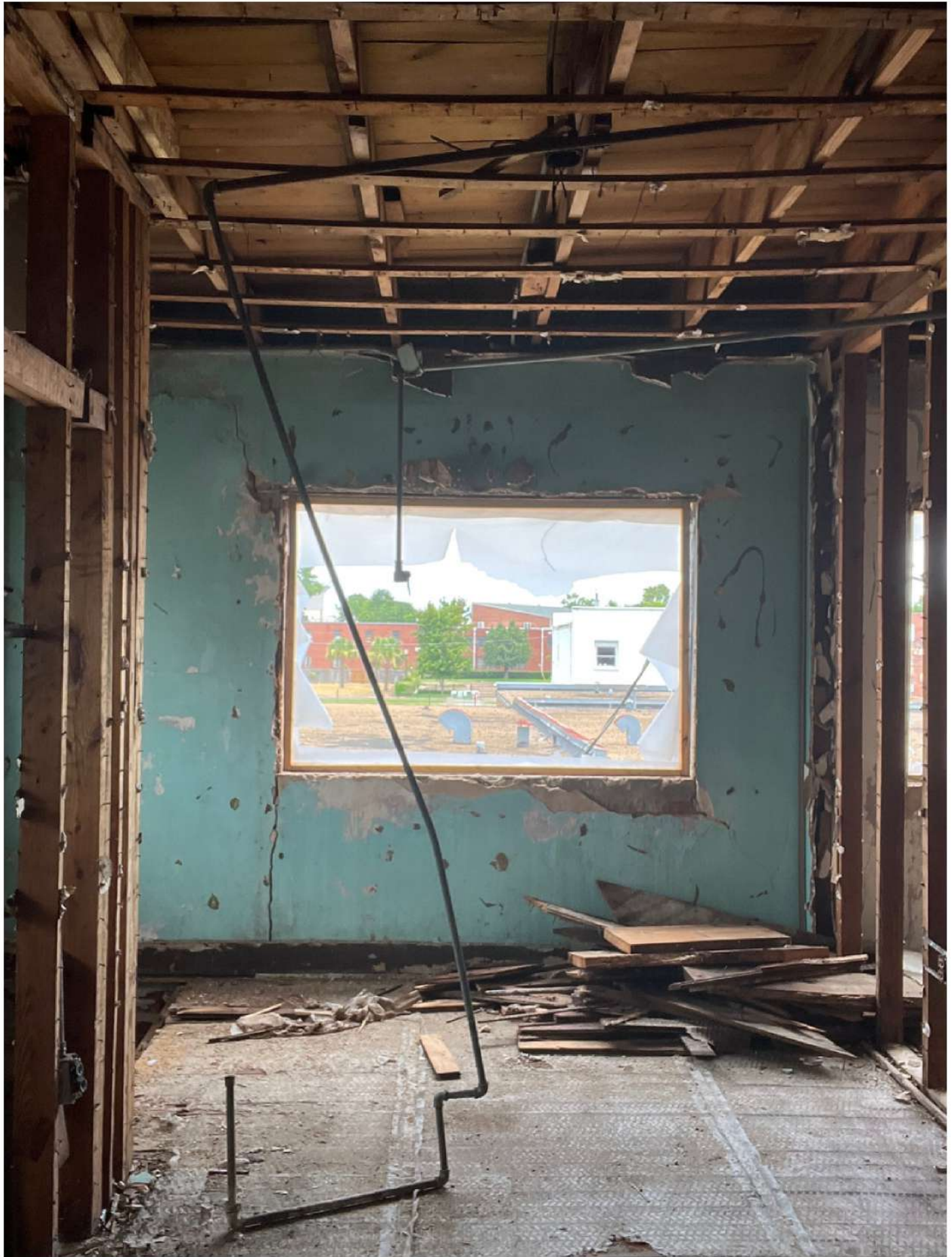
Interior-Space 15 Farish Street Building 2nd Level (YWCA Side)
