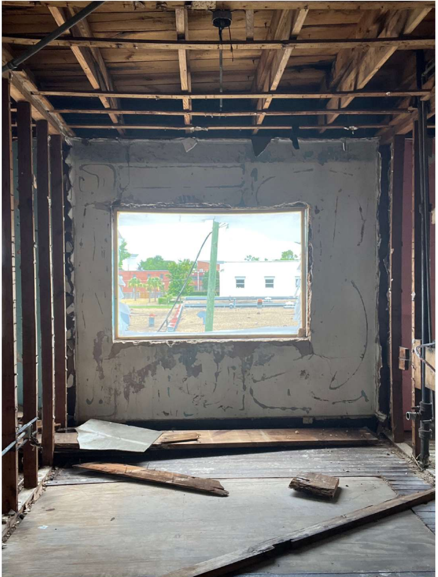
Interior-Space 13 Farish Street Building 2nd Level (YWCA Side)
