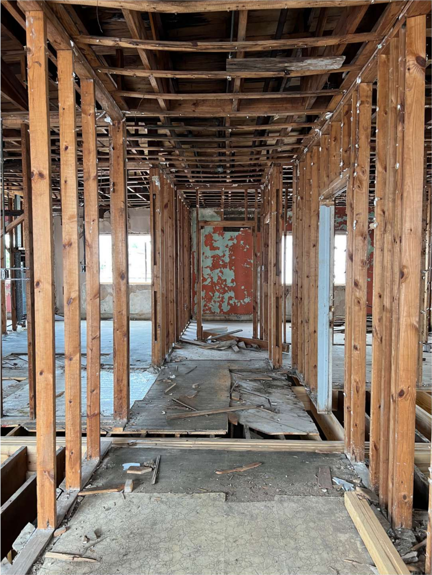
Interior-Upstairs Hallway Leading From Street Level Staircase
