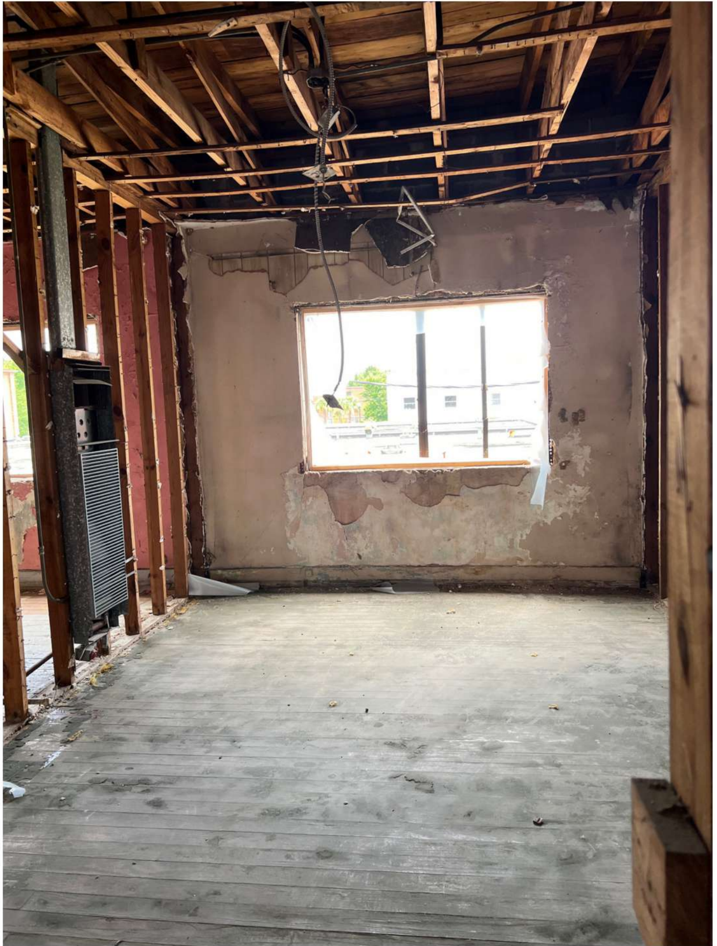
Interior-Space 9 Farish Street Building 2nd Level (YWCA Side)
