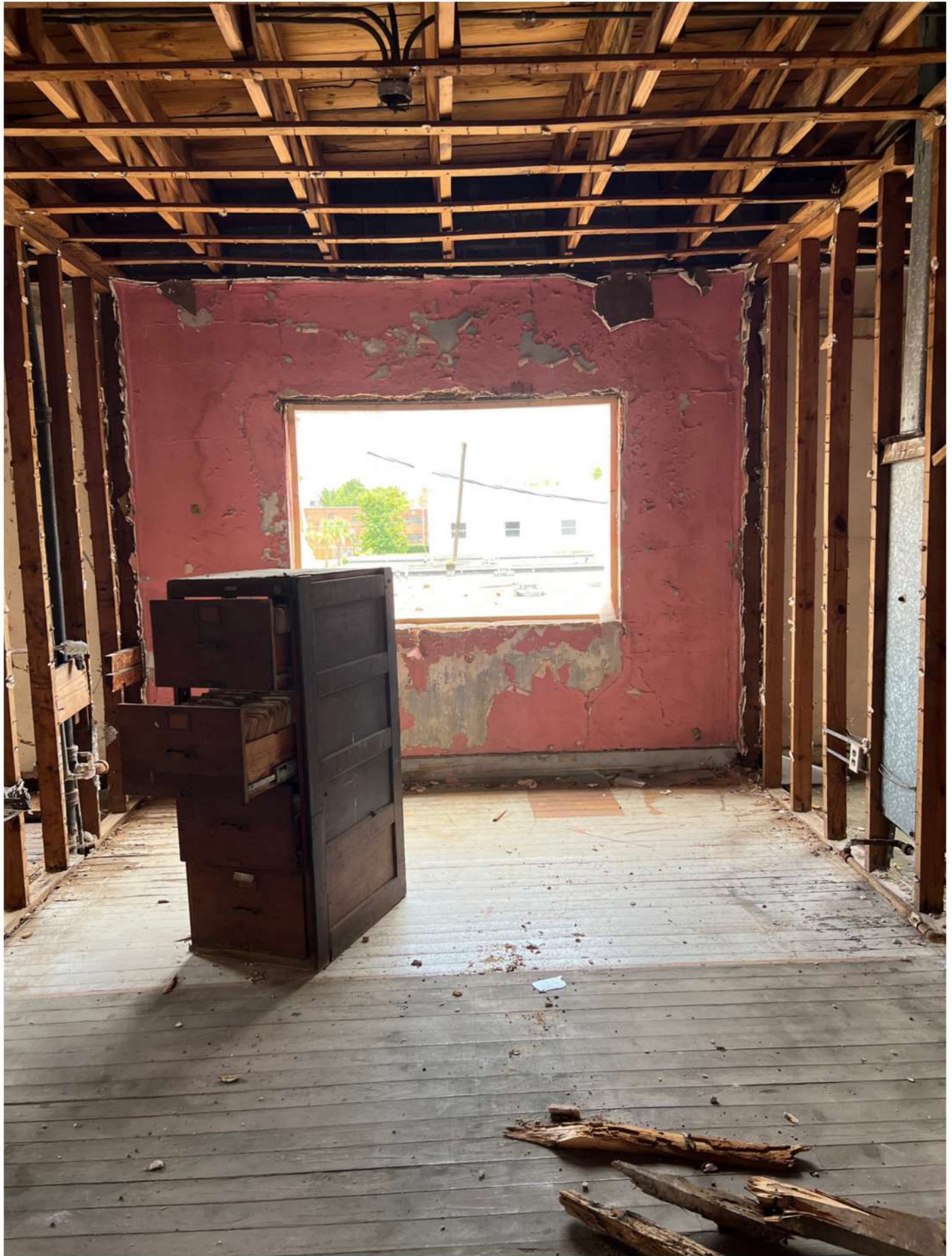
Interior-Space 11 Farish Street Building 2nd Level (YWCA Side)
