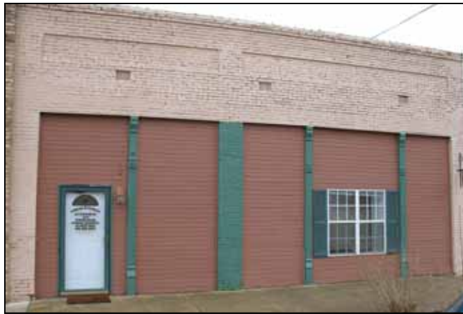
This historic commercial building in Como, Mississippi has been drastically altered with the removal of the original display glass and doors and replacement with inappropriate wood siding and a modern residential style door and windows. The original cast iron columns are still visible showing the original divisions of the storefront.
