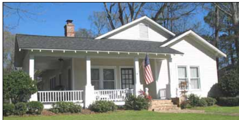
This Craftsman style house at 217 West Main Street has a projecting porch with tapered columns on brick piers typical of that style.
