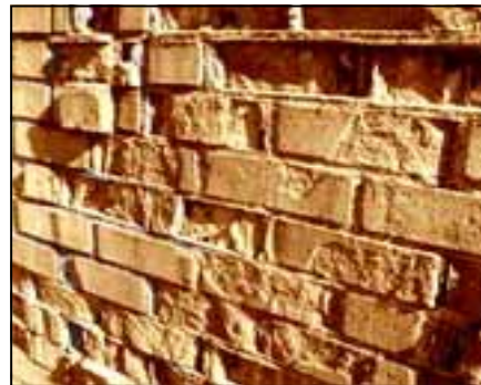
This photograph supplied by Chagrin Falls Preservation in Ohio illustrates the spalling that can occur only five years after using portland cement mortar in repointing.
