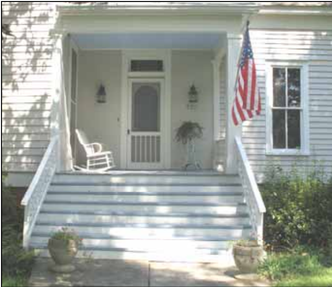
The steps of this Queen Anne style house at 237 North Oak Street are appropriately constructed of wood.
