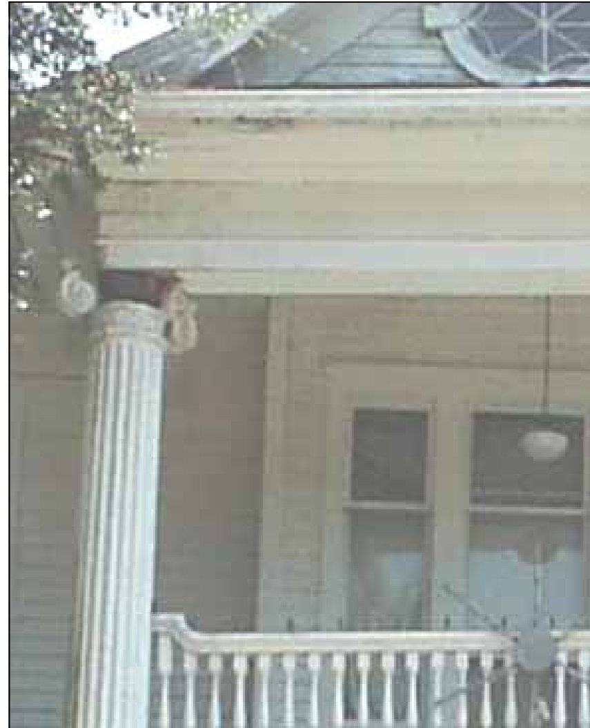
Failure to clean and maintain gutters is the primary cause of porch deterioration such as the damage caused to the column capital.
