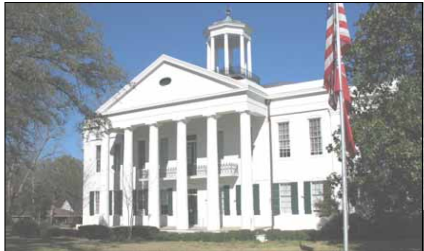
The Courthouse has typical Greek Revival characteristics such as rectangular massing, low pitched roof, Grecian Doric columns without bases, and stucco scored to look like stone.
