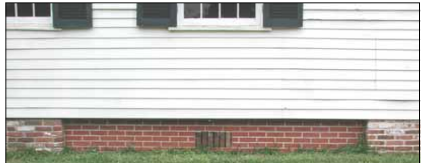
At least this homeowner recessed the new brick crawl space enclosure. This treatment would look more appropriate if the new brick were painted black and faced with lattice.
