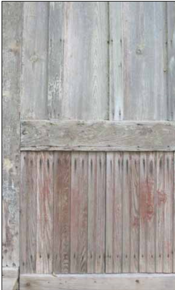
The Raymond railroad depot uses a combination of board-and-batten siding over tongue-and-groove beadboard siding.
