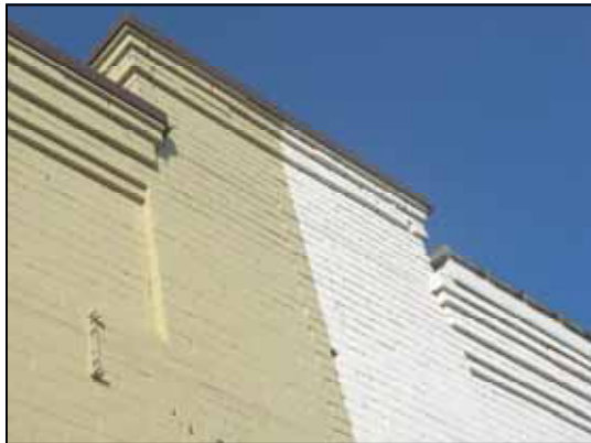
The brickwork of the parapets on several commercial buildings in Raymond feature decorative brick patterning and projecting bricks to give interest to the façade.
