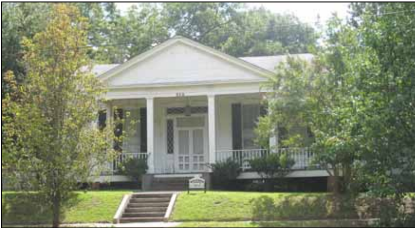
The house at 214 Port Gibson Street is Greek Revival in style with its gabled projecting porch supported on square vernacular columns and typical multi-paned windows.
