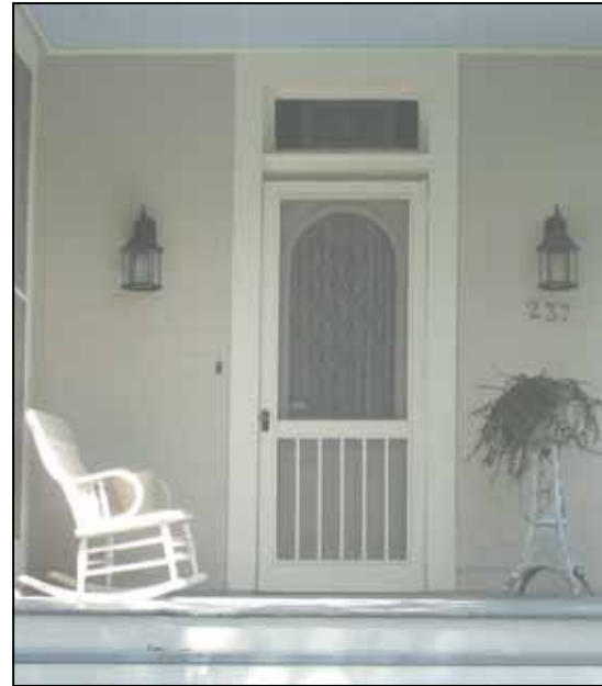
The screen door of this Queen Anne style house at 237 North Oak Street is most likely a later addition, however it is simple in design and properly fits the door opening.
