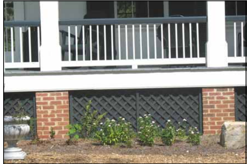
The lattice panels between the brick piers appropriately enclose this crawl space.
