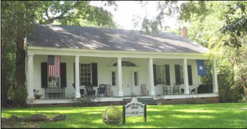
104 Dupree Street has a low-pitched side gable roof which is typical of the Greek Revival style.
