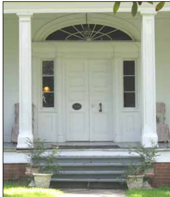
The steps of this Greek Revival style house at 104 Dupree Street are appropriately constructed of wood painted the same color as the porch floor.
