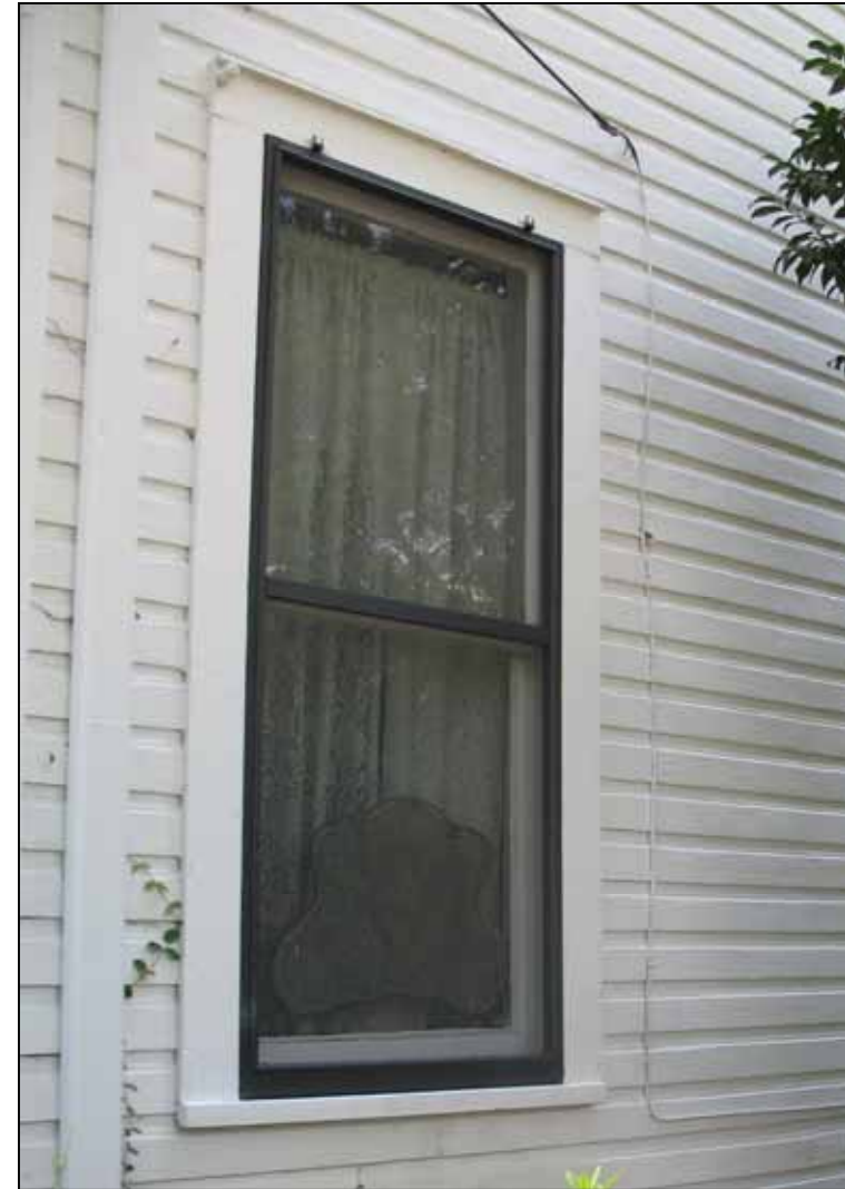
The house at 101 Dupree Street uses Shiplap siding on the side of the house.
