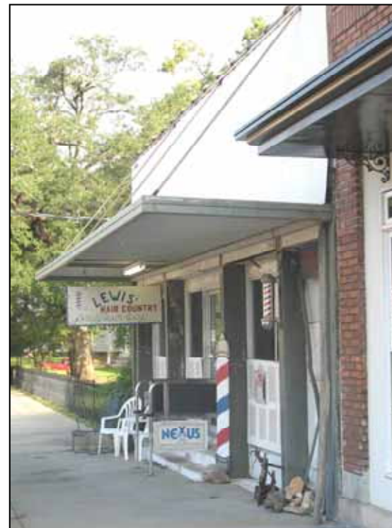
117 West Main Street uses a suspended metal canopy supported by metal rods which was very common for commercial buildings built in the 1910s to 1940s. Several buildings on East main Street still have visible hooks on the front walls where the canopy supports were attached.
