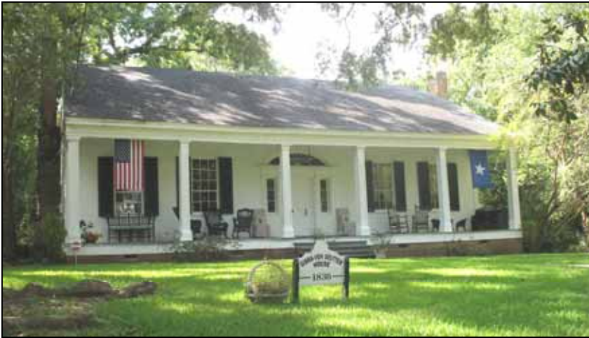
104 Dupree Street has a full width inset gallery supported on square vernacular wood columns, and a low-pitched roof typical of the Greek Revival features.
