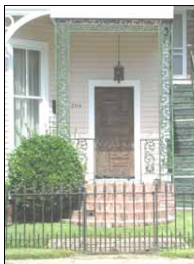
This Queen Anne style house has lost its original corner porch and entrance doorway. The original doorway would have featured a transom and single-leaf door with glazed upper panel. The original porch was enclosed and a new, inappropriate 1970s door with raised panels was installed. Unfortunately, the house also lost its original porch detailing and entrance steps.
