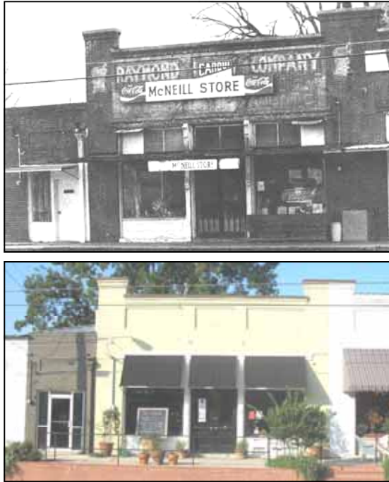
The top photo (courtesy of Pattie Adams Snowball) shows 104 East Main Street in the 1940s and the bottom photo is the same building today. The building is a store-front type with a central entrance flanked by display glass and separated by cast iron columns. Note the original transoms in the top photo which are now covered by the awning. Originally the building had a suspended metal canopy rather than the awnings it has today.
