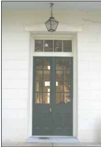
The Courthouse has a stucco finish which is scored to look like stone blocks, a characteristic of the Greek Revival style.
