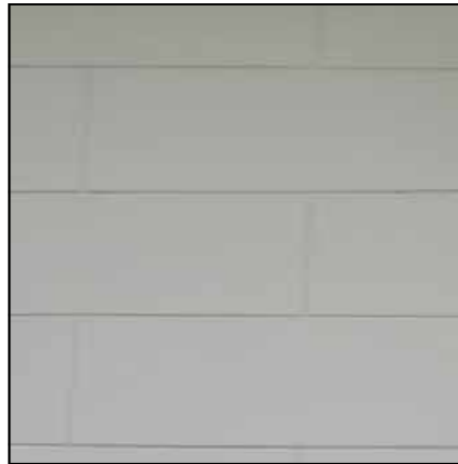
The Courthouse has a stucco finish which is scored to look like stone blocks, a characteristic of the Greek Revival style.
