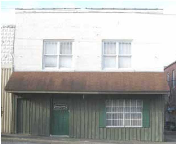
This historic commercial building in Newton, Mississippi had an inappropriate shingled awning added to the building and the original storefront was removed and inappropriately replaced with board-and-batten siding with a residential door and windows.
