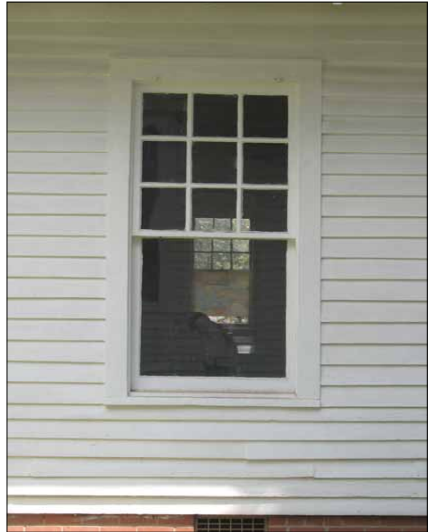
125 Port Gibson Street uses beveled wood siding which is typical of the Craftsman style of architecture.
