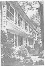
Greenbrier's window and doorway overhungs are lined with pressed wood which was also used as shouthing in the construction of the house. It's moisture-resistant, devable
