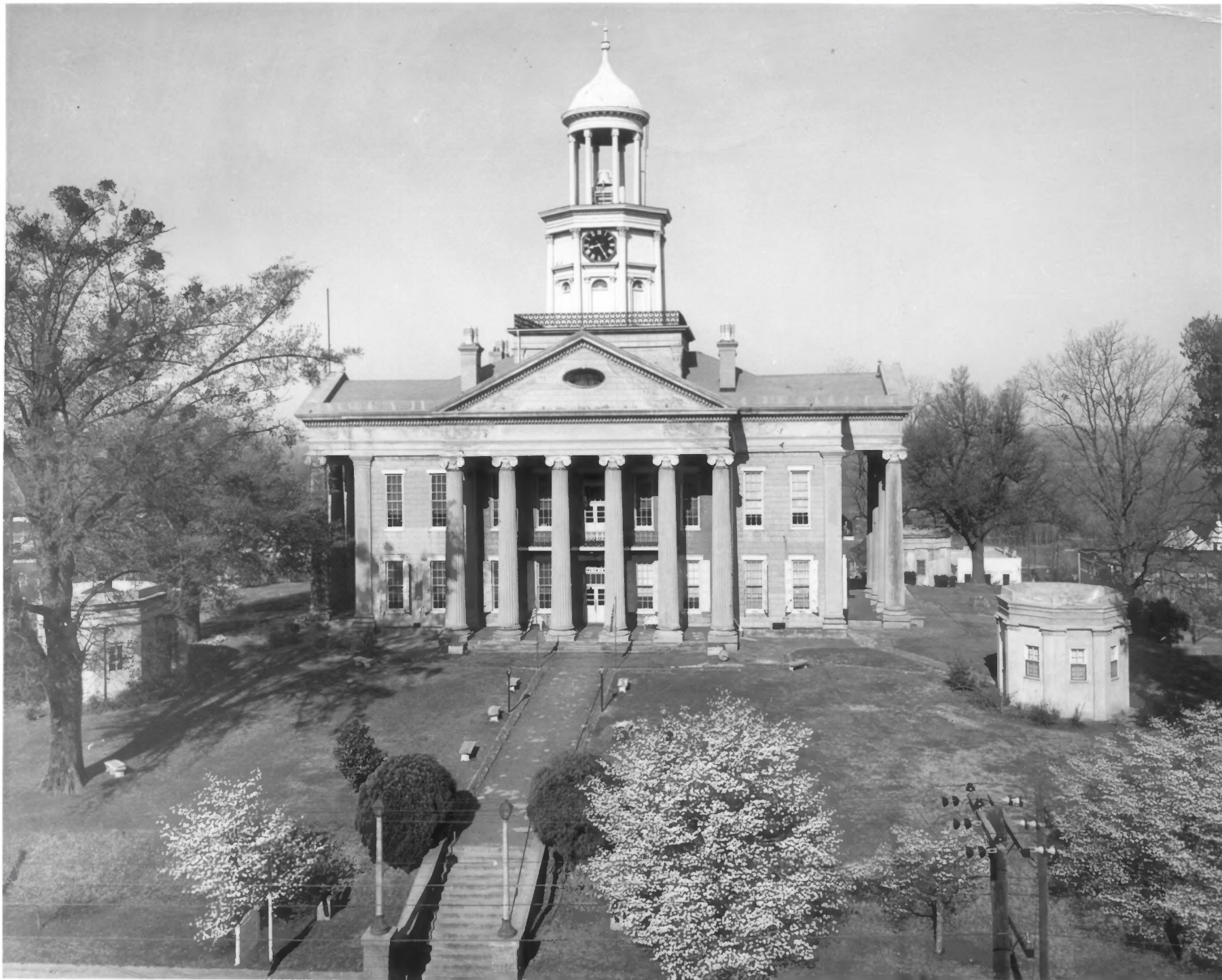
Old Warren County Court House, Vicksburg, Mississippi
